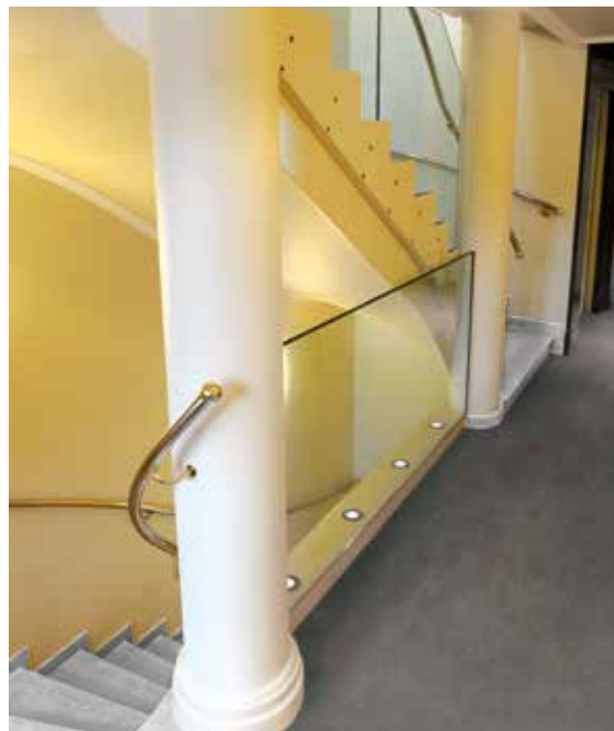
Glazed railing and mirror polished stainless steel handrail | Hotel Cours d'Alsace, France
