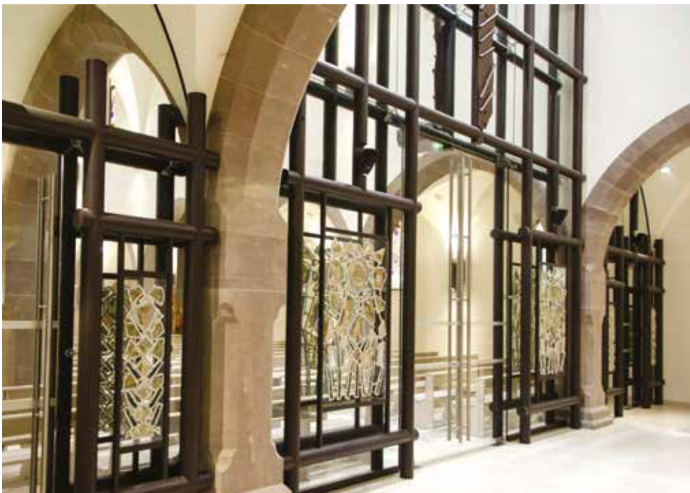
Separation wall, stapled glazing, church renovation Strasbourg - France
